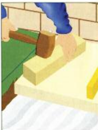
▲ (fig. 5) The slab can be gently tapped until they are the correct level.
