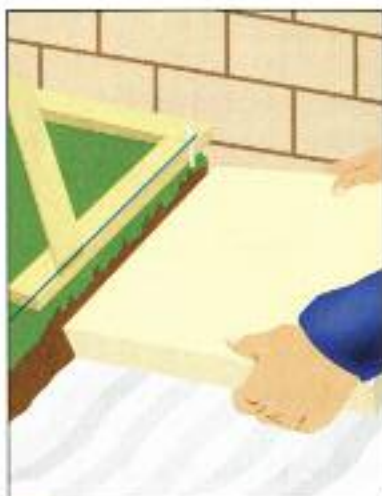
▲ (fig. 4) Before the first slab is laid, check the string guidelines are square to the house using the builder's square.
