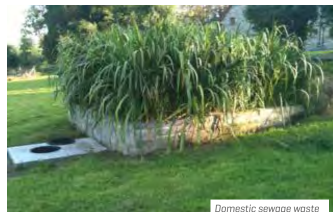
Domestic sewage waste treatment system.
