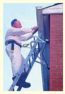
Microlite and ladder belt restraint in use
