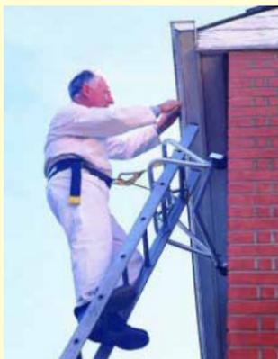
Microlite and ladder belt restraint in use.
