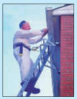
Microlite and ladder belt restraint in use
