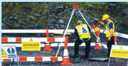
Preparing for a safe confined space entry
