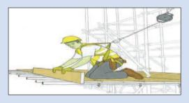
Scaffolder using a harness and inertia reel
